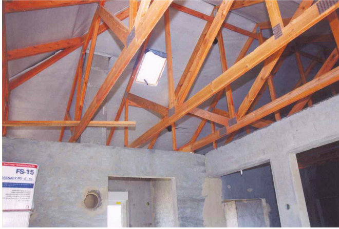
Fig. 4. The internal structure of the building.
