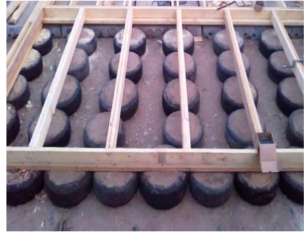
Fig. 4. The foundation of a building from automobile tires
