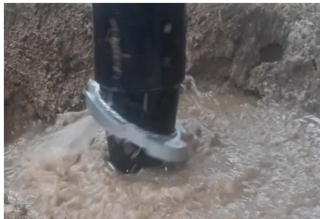
Figure 7 – Drilling process at high speeds of the drilling tool
