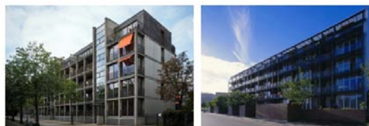
Figure 1. Germany. Reconstructed large-block residential buildings [10]
