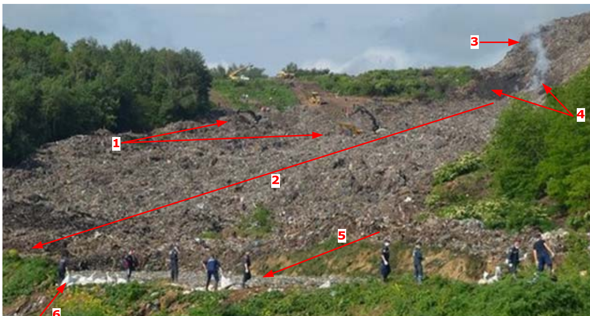
Figure 1 – Emergency work for the decommissioning of the SW landfill:
