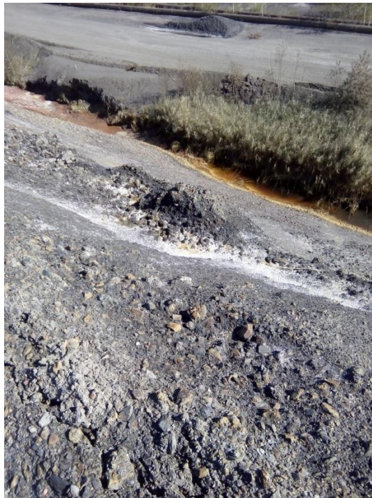
Fig. 1 - Sulfate waters at the foot of the dump of the coal-preparation plant of the Lviv Coal Company PJSC
