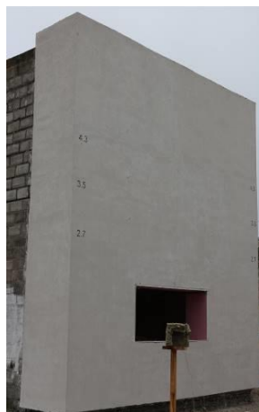
Figure 2. Appearance of a fragment of a building to be used for testing of external wall constructions fit with façade heat insulation and finished with rendering and heat insulating material for fire spread before commencement of the tests
